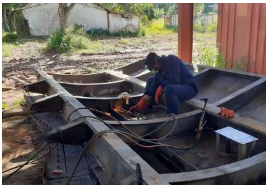
Figure 8-5: Fabrication and installation of Kudawilachchiya Radial Gates
