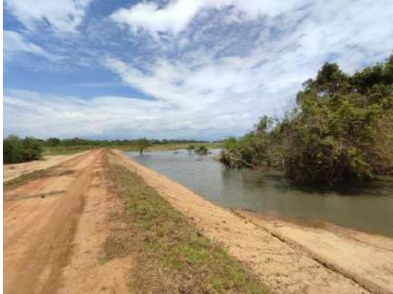
Figure 5-29: Construction of Mankada wewa
