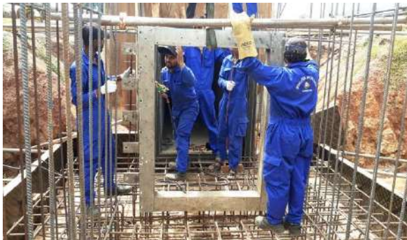
Figure 8-7: Sluice gate fabrication and installation of Lower Malwathu Oya Project by Regional workshop Rambewa
