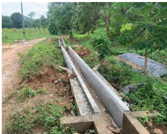
Figure 6-12: Construction 171 m long canal lining in FC 3 in Elahera division
