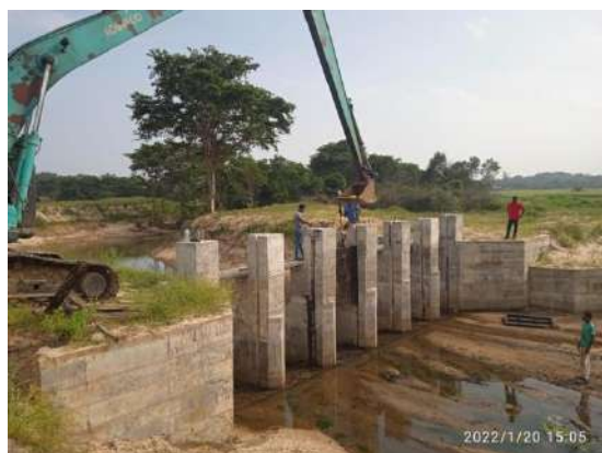
Figure 8-2: Fabricate and installation of Bomiriya flood control Anicut gates at Kaduwela
