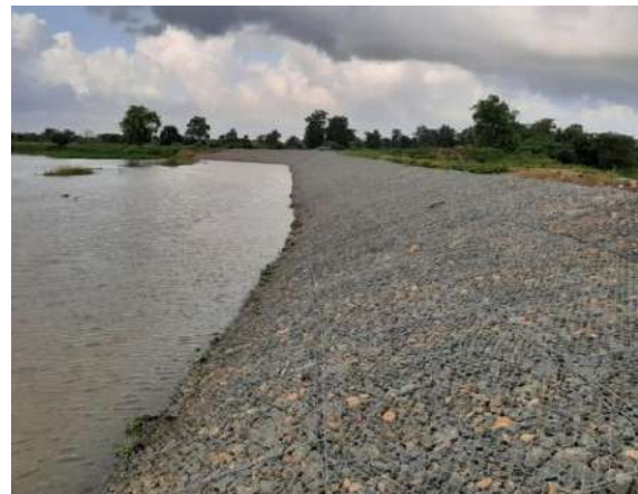
Figure 7-6: Improvements to Naathanodai flood protection bund from 0+270 to 0+360
