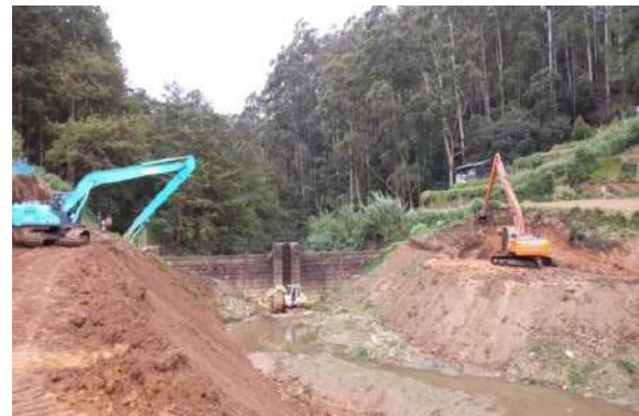
Figure 5-28: Excavation & removal of silt
