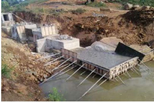
Figure 5-11: Construction of Sluice Structure
