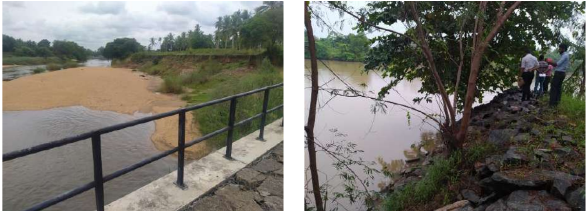
Figure 4-25: Field inspection for Maa Oya and Deduru Oya
