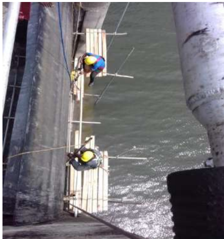
Figure 8-21: Repair and installation of cables to Hakwatuna Oya radial gates
