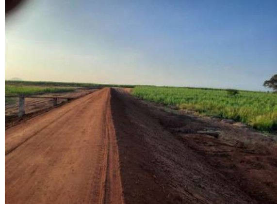
Figure 5-30: Meepale Tank Improvements
