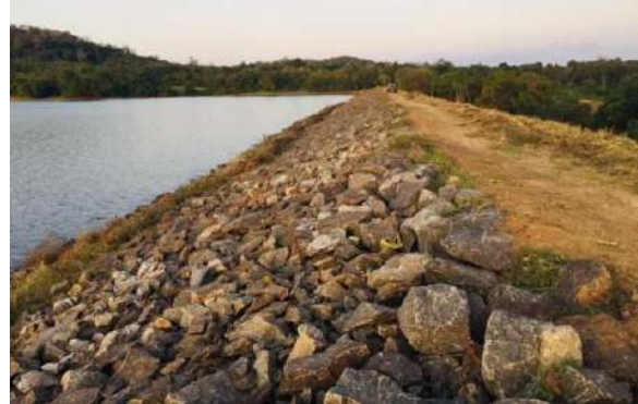
Figure 6-21: Bibila Badulu Oya after Rehabilitation
