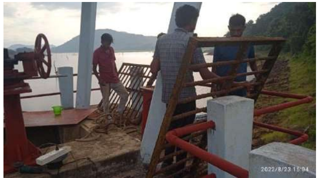
Figure 8-4: Repairing of Pannalgama Sluice gate and trash rack at Ampara
