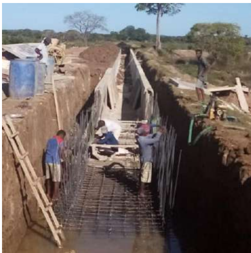
Figure 5-2: Issanwewa Main Canal
