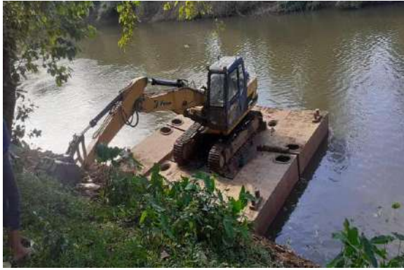
Figure 7-2: Clearing obstacles along the Nilwala River from Akuressa to Pitabeddara
