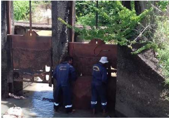
Figure 8-13: Kahagaha Amuna Gate repair at Weeraketiya
