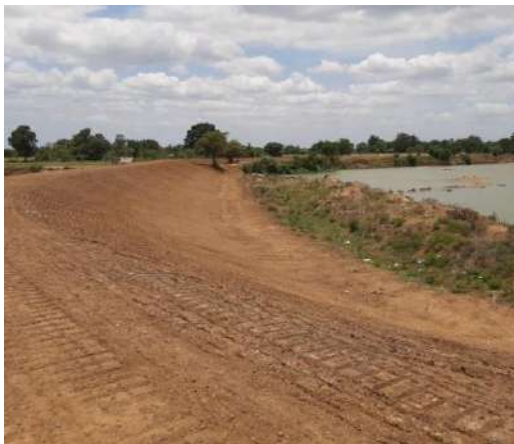
Figure 7-6: Improvements to Naathanodai flood protection bund from 0+270 to 0+360
