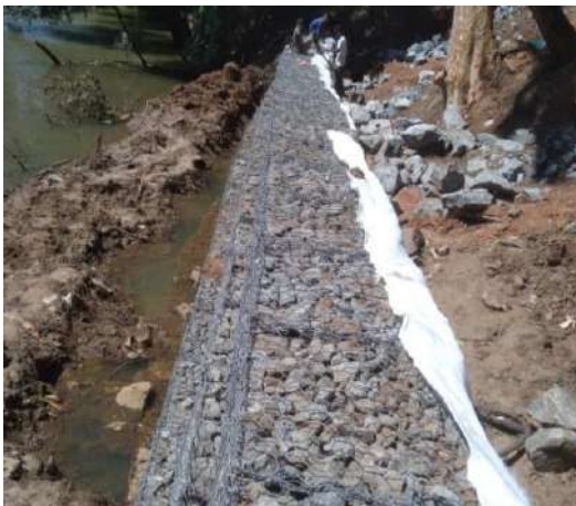
Figure 7-5: Construction of Gabion wall at Bolana in Walawa River Left bank
