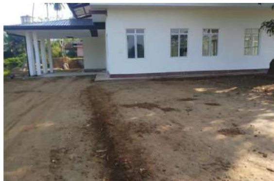
Figure 5-5: Construction of Project Director's Office
