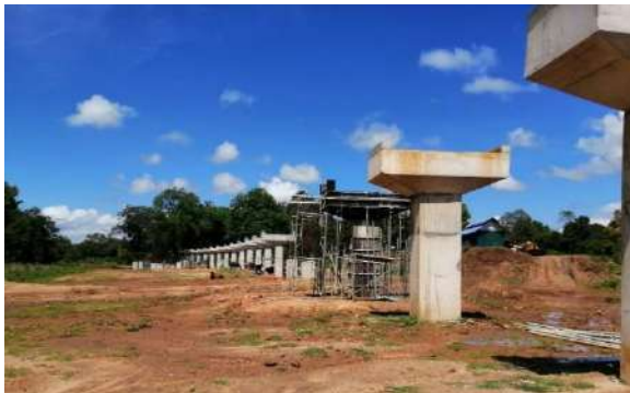
Figure 5-16: Kuda Oya Transfer Canal
