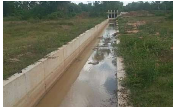
Figure 5-10: Spill tail canal of Walanthaliyawa Tank
