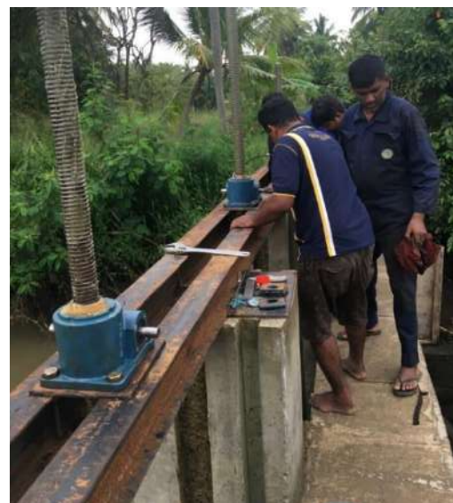
Figure 8-22: Repair and installation of hoisting arrangements of Thanthuneriya main channel
