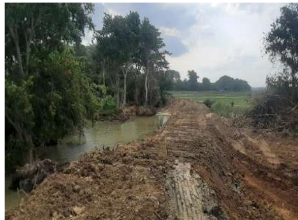
Figure 7-9: Clearing Drainage Canals – Ampara
