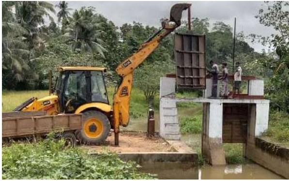
Figure 8-10: Weni Akula anicut gates fabrication and installation by Regional workshop Halpathota
