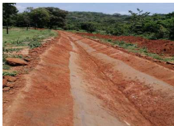
Figure 5-21: Construction of FC 01
