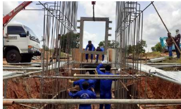
Figure 8-7: Sluice gate fabrication and installation of Lower Malwathu Oya Project by Regional workshop Rambewa
