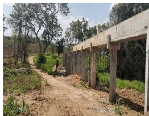
Figure 5-25: Construction of Structures
