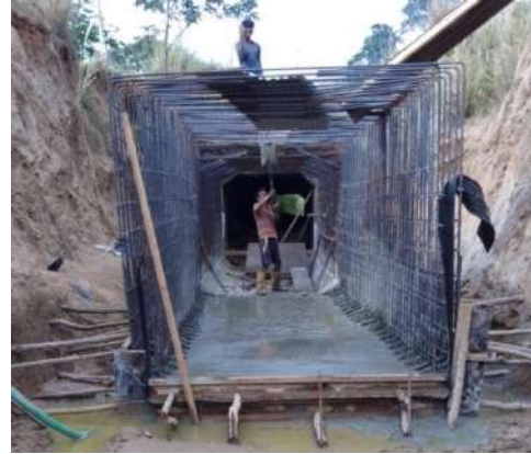
Figure 5-27: Construction of closed Conduit structure
