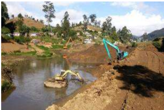
Figure 5-28: Excavation & removal of silt
