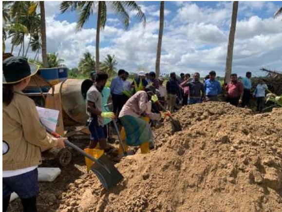
Figure 4-12: Stock piled soil for Canal road construction
