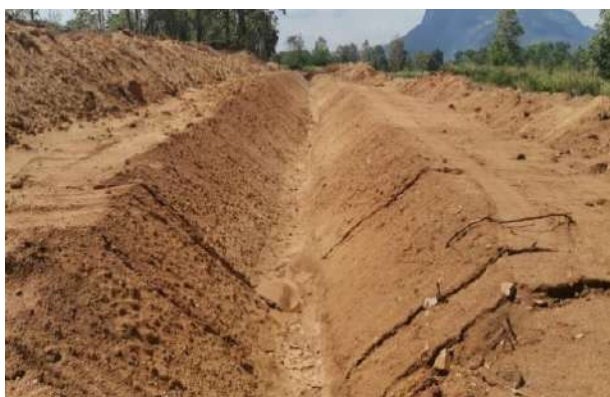
Figure 5-24: Construction of Main canal
