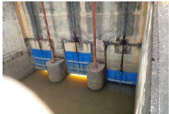
Figure 8-8: Thalгахagoda Gravity gates fabrication and installation
