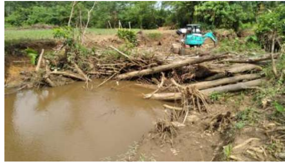
Figure 7-11: Clearing Drainage Canals – Ambalangoda (Bentara Ganga Basin)
