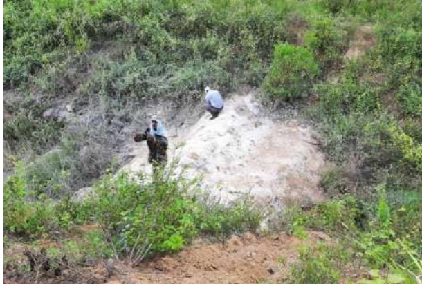
Figure 5-26: Rock blasting work
