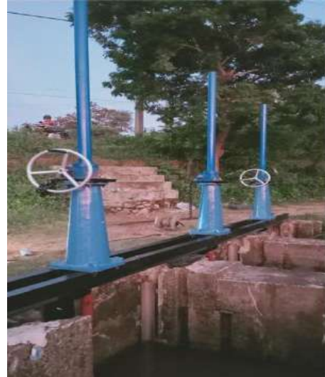
Figure 8-23: Repair and installation of hoisting arrangements Mavil aru LB & RB channel
