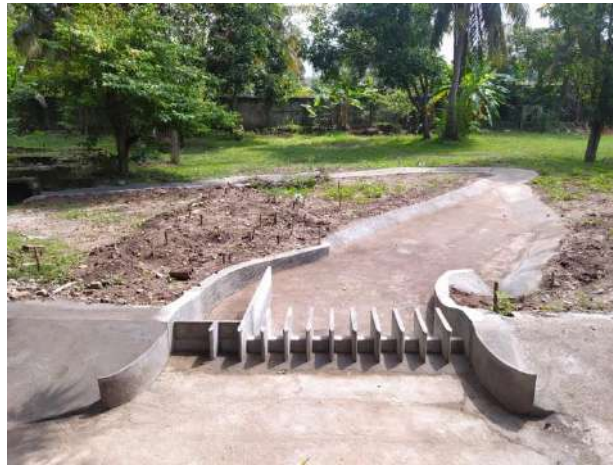
Figure 4-24: Model construction of Lower Malwathu Oya reservoir
