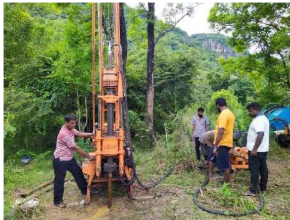
Figure 4-18: Geotechnical Investigation at Kotapathdamana Tank
