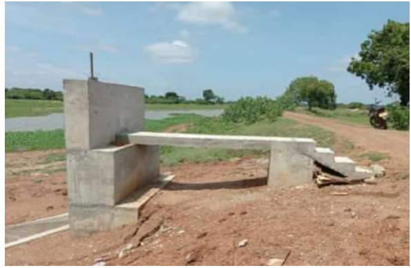
Figure 6-15: Murugan Kulam after Rehabilitation
