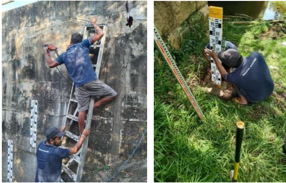
Figure 4-5: Installing Gauge Posts under the Wewgam Pubuduwa Project
