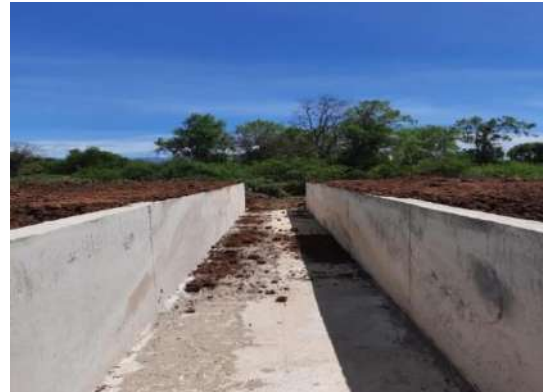
Figure 5-19: Construction of Debara Ara feeder canal
