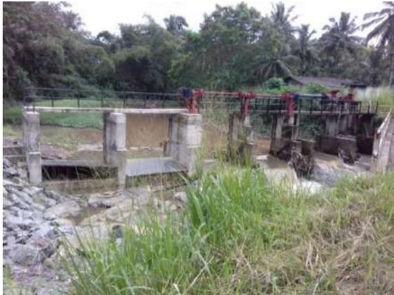
Figure 8-20: Fabrication and installation of collapsible flap gates at Wilgoda anicut
