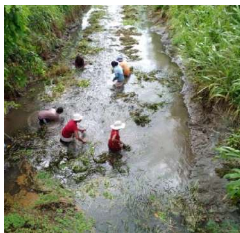
Figure 7-7: Removing aquatic plants along Neelabemma feeder canals in Neelabemma scheme
