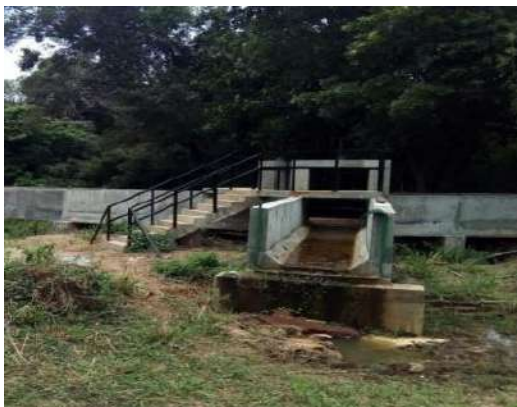
Figure 5-20: Construction of RB Canal
