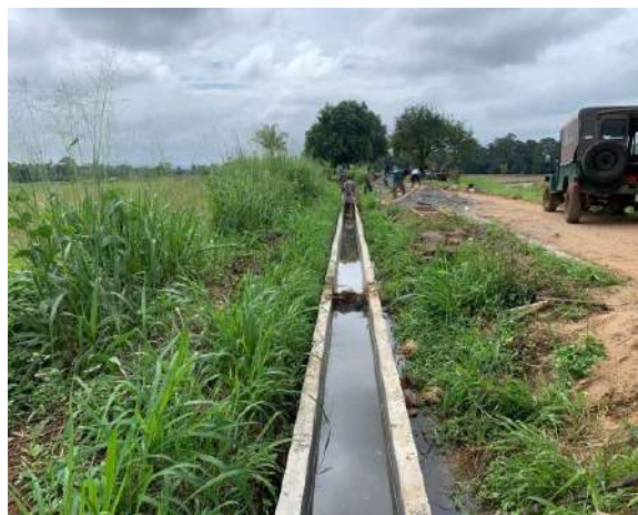
Figure 6-13: Construction 180 m lining in FC 14 Akkara 200 in Elahera division
