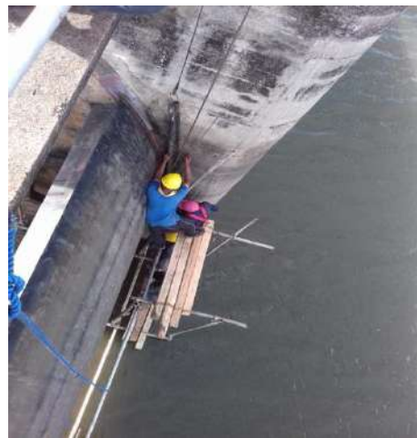
Figure 8-21: Repair and installation of cables to Hakwatuna Oya radial gates
