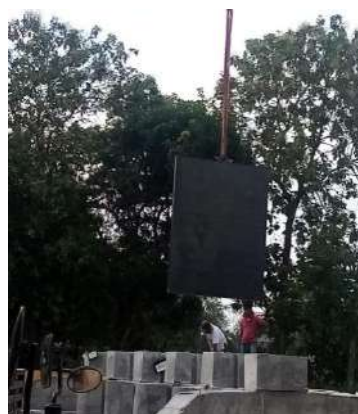
Figure 8-2: Fabricate and installation of Bomiriya flood control Anicut gates at Kaduwela
