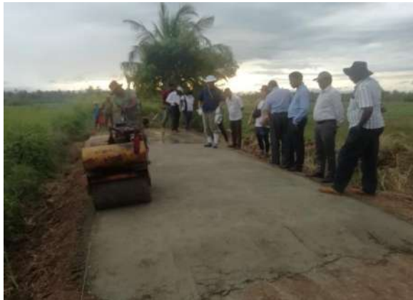
Figure 4-14: Compaction by 1 ton roller in the road construction
