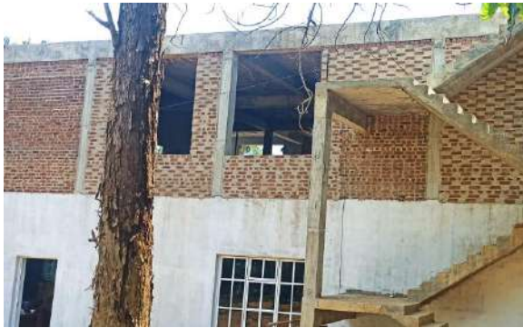
Figure 5-6 Construction of office building for the PMU
