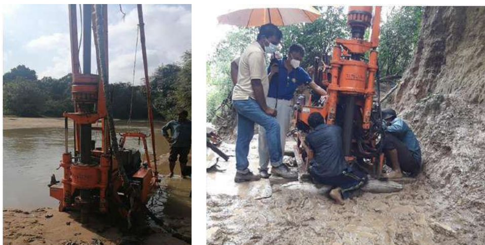
Figure 4-17: Geotechnical Investigation works at Balagala tank
