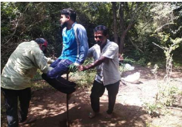
Figure 4-6: Augering in Pan kulam Aru Reservoir bed
