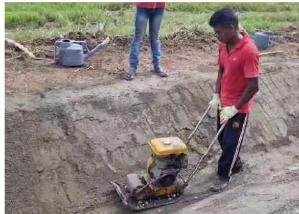
Figure 4-15: Compaction by Plate Wacker in canal lining
