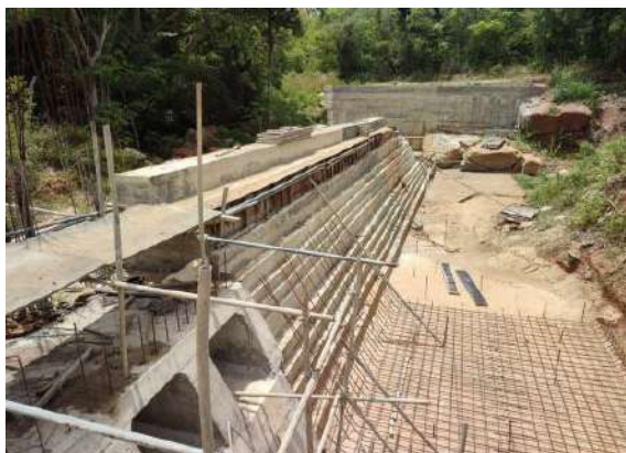
Figure 5-22: Construction of Anicut
