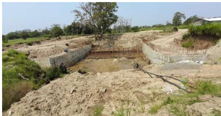
Figure 5-33: Construction stage of Pan Oya Anicut
