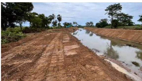
Figure 7-10: Clearing Drainage Canals – Batticaloa
