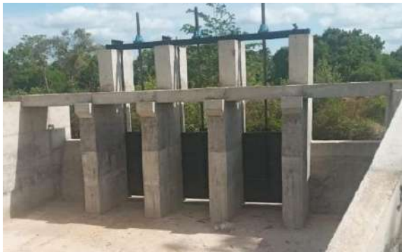
Figure 5-9: Spill gates of Walanthaliyawa Tank
