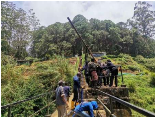
Figure 8-19: Barak plain Tank sluice repair
