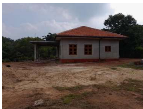
Figure 6-10: Construction of Morawewa Unit Office in Trincomalee Region
