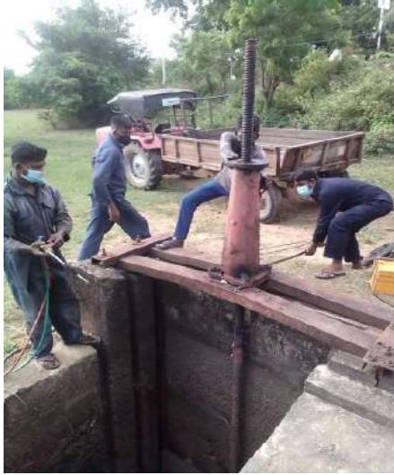
Figure 8-23: Repair and installation of hoisting arrangements Mavil aru LB & RB channel
