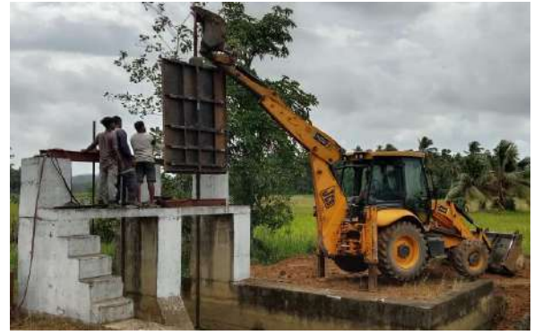
Figure 8-10: Weni Akula anicut gates fabrication and installation by Regional workshop Halpathota
