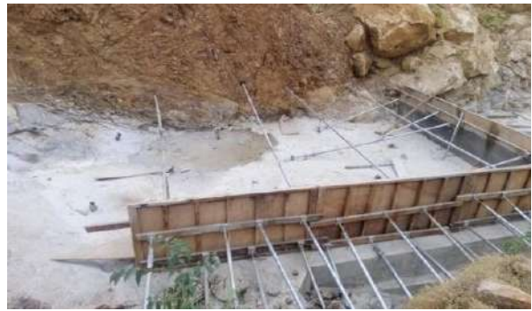
Figure 5-12: Construction of Saddle Dam
