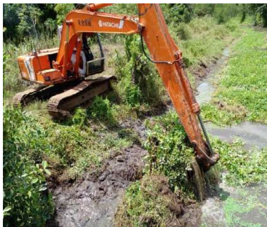
Figure 7-7: Removing aquatic plants along Neelabemma feeder canals in Neelabemma scheme
