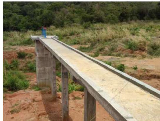
Figure 5-23: Construction of LB Sluice
