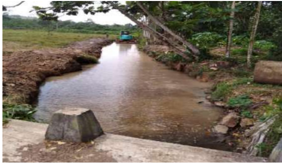
Figure 7-11: Clearing Drainage Canals – Ambalangoda (Bentara Ganga Basin)
