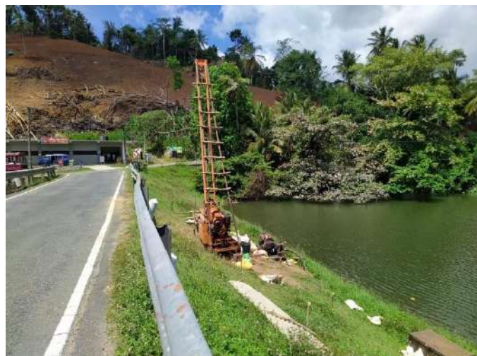
Figure 4-19: Foundation Treatment works at Denagama Tank
