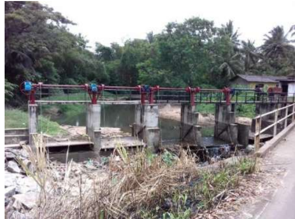
Figure 8-20: Fabrication and installation of collapsible flap gates at Wilgoda anicut
