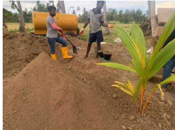
Figure 4-13: Stock piled soil after removing soil lumps and after drying up
