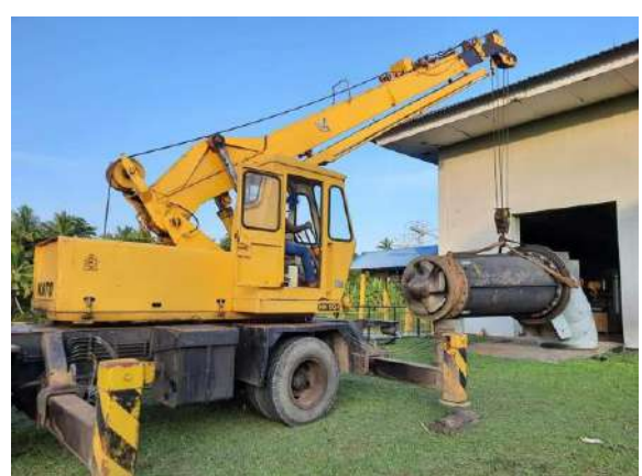
Figure 8-12: Overhauling axial flow pump at Magallagoda Pump house
