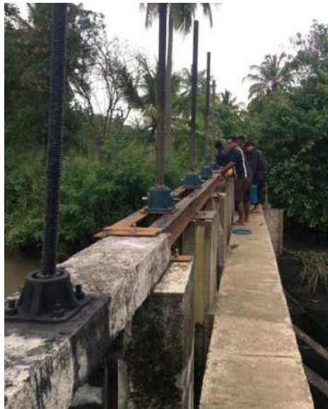
Figure 8-22: Repair and installation of hoisting arrangements of Thanthuneriya main channel
