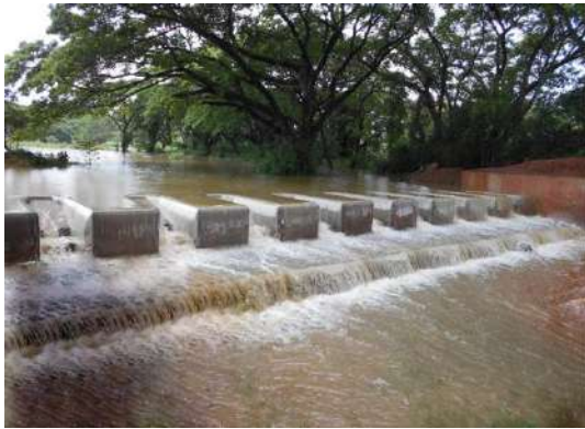
Figure 5-18: Construction of Debara Ara feeder canal
