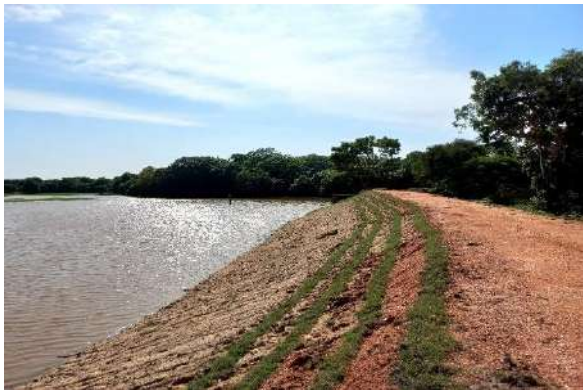
Figure 6-16: Maha Wewa after Rehabilitation
