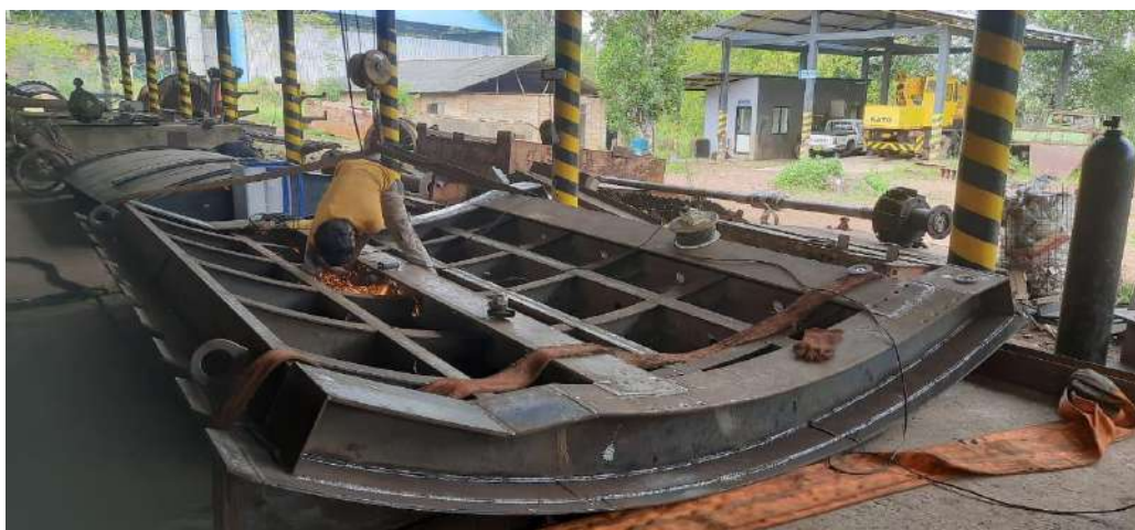
Figure 8-9: Handapanagala pickup anicut gates fabrication
