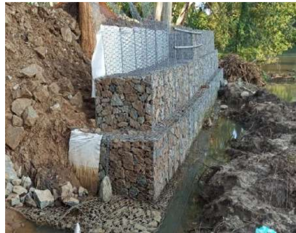
Figure 7-5: Construction of Gabion wall at Bolana in Walawa River Left bank
