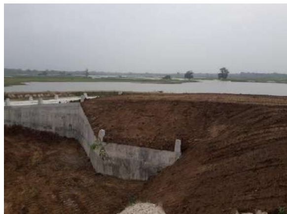
Figure 11-116: Mavil Aru 1000ft Causeway after Construction
