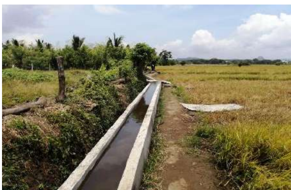
Figure 11-76: Canal system improvement in Puwakpitiya, Dambulla Division
