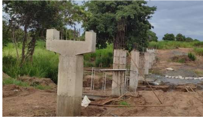
Figure 11-24: construction of D canal trough extension of Wilakandiya project
