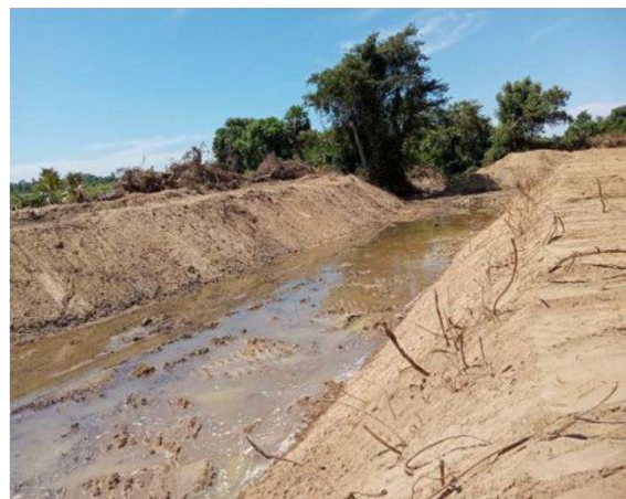
Figure 11-35: Widening and straightening in Mavalai River
