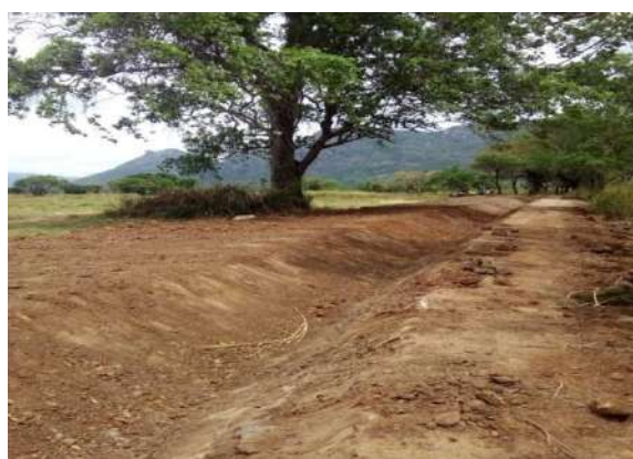
Figure 11-67: Construction of field canals
