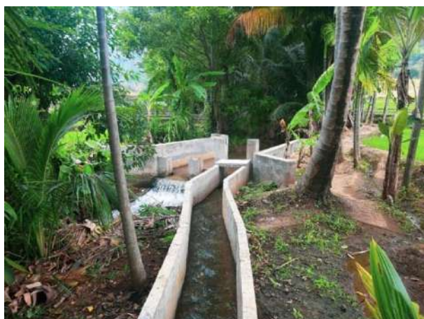
Figure 11-27: Iththanilla kandura anicut and canal lining
