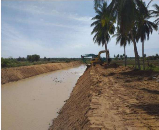
Figure 11-34: Widening & straightening of Karavetti river
