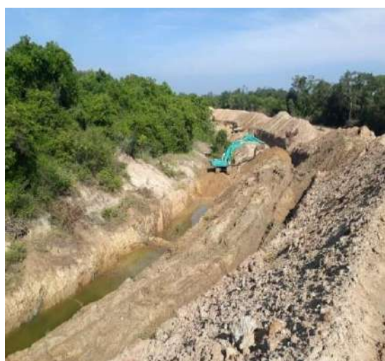
Figure 11-15: construction work of feeder canal
