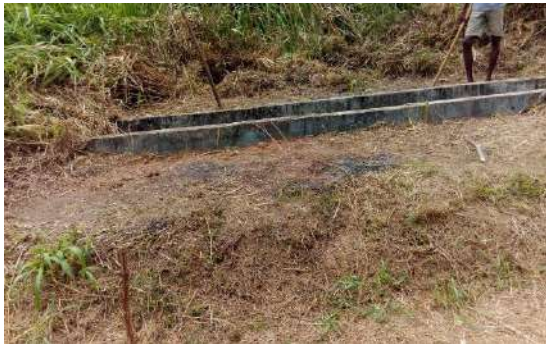
Figure 11-57: Before the construction of Tractor crossing
