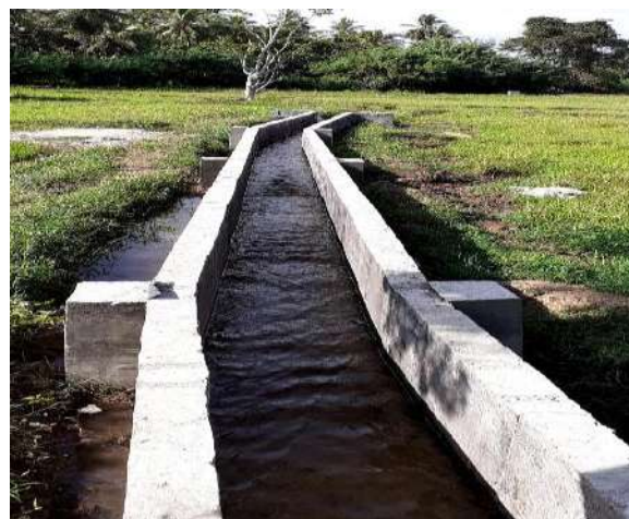
Figure 11-89: Canal lining of Yakadapotha Tank in Wariapola Division
