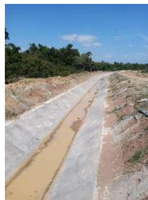
Figure 11-14: Issanwewa D Canal lining
