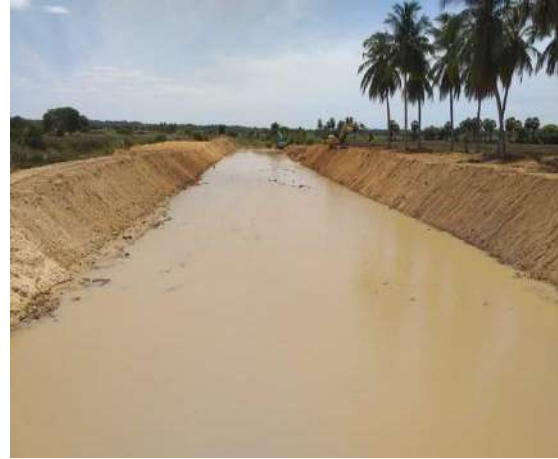
Figure 11-34: Widening & straightening of Karavetti river
