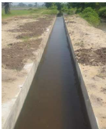
Figure 11-110: Construction of canal lining in Eluwankulam Scheme
