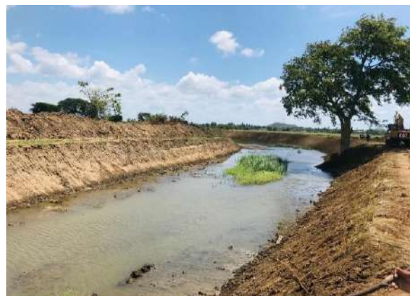
Figure 11-120: Kanthale Spill Tail Canal after Construction
