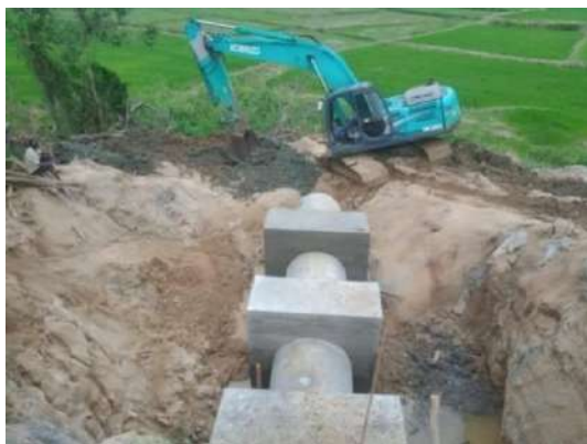
Figure 11-3: Construction of Morning glory spillway
