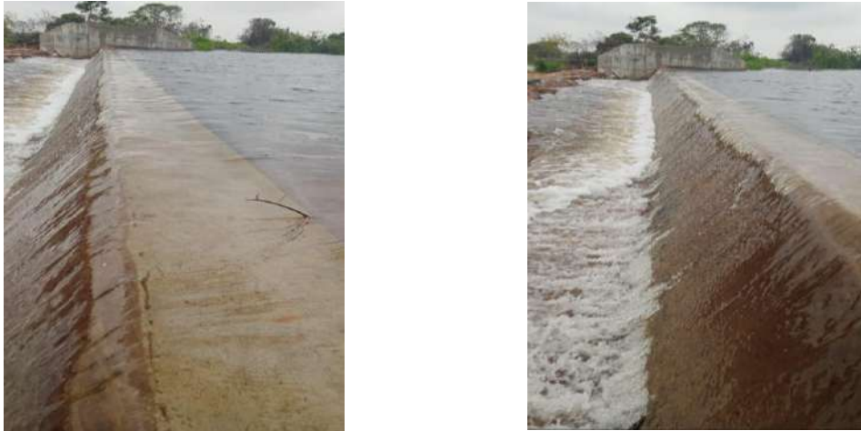
Figure 11-112: Construction of Spill structure for Bogahawewa in Inginiyitiya Division
