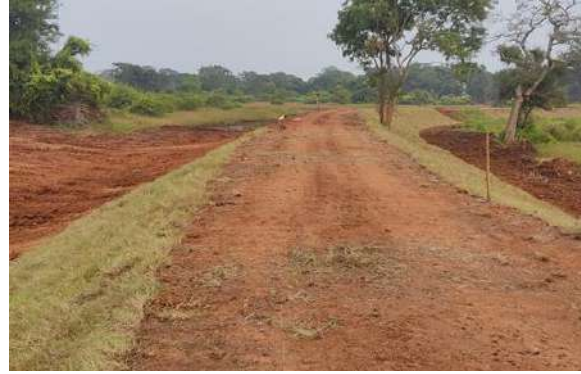
Figure 11-19: Rehabilitation of Diulgahawewa Tank
