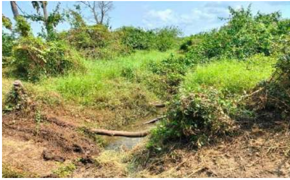
Figure 11-117: KottalAru Drainage Channel before Construction
