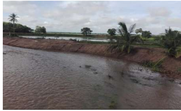
Figure 11-118: KottalAru Drainage Channel after Construction
