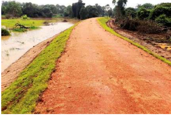
Figure 11-18: Rehabilitation of Palugollewa Tank
