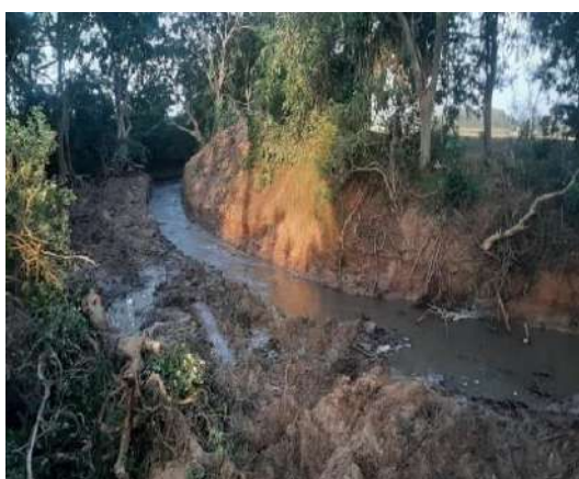
Figure 11-6: Maintenance of Drainage Canals of Kunchanodai Anicut
