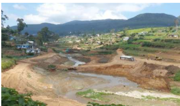
Figure 11-70: Desilting work at Barrack plane tank
