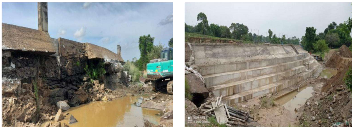
Figure 11-36: Reconstruction of D/S spillway (LB) in Unnichchai tank
