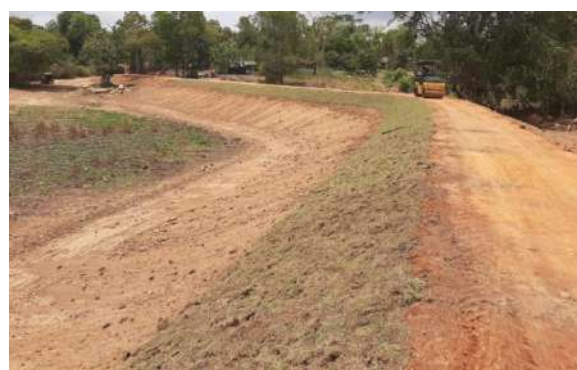
Figure 11-91: Bulnewa Tank, Galgamuwa Division
