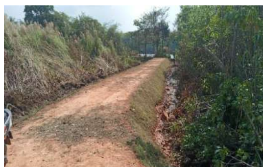
Figure 11-48: After the improvements to Kahaunage MFP bund
