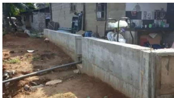
Figure 11-50: After the construction of flood protection wall at Pattiwala
