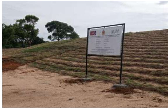
Figure 11-128: Olugollawa Wewa after Rehabilitation
