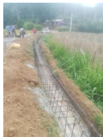
Figure 11-28: Panangala main canal
