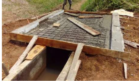
Figure 11-58: During the construction of Tractor
