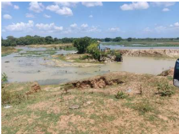
Figure 11-115 : Mavil Aru 1000ft Causeway before Construction
