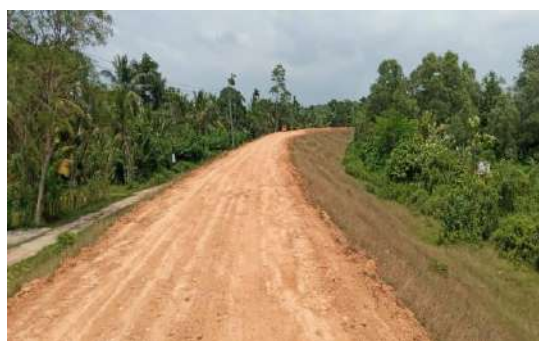
Figure 11-47: Bolgoda bund after gravelling
