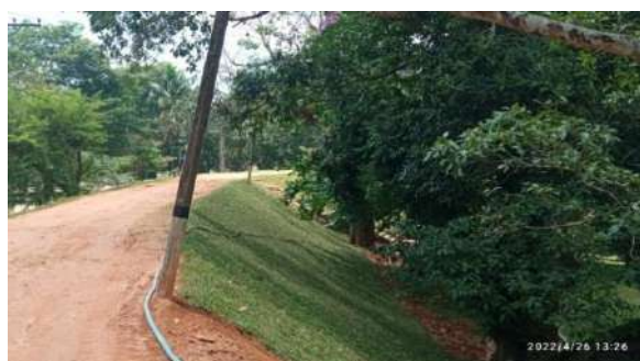
Figure 11-49: After the improvements in Kelani north bund from 5+530 to 6+050
