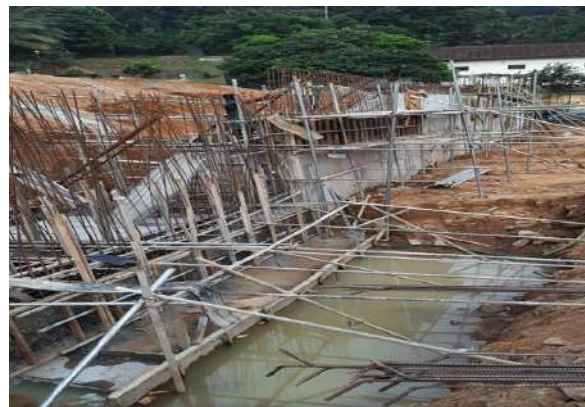
Figure 11-72: Construction work of retaining wall
