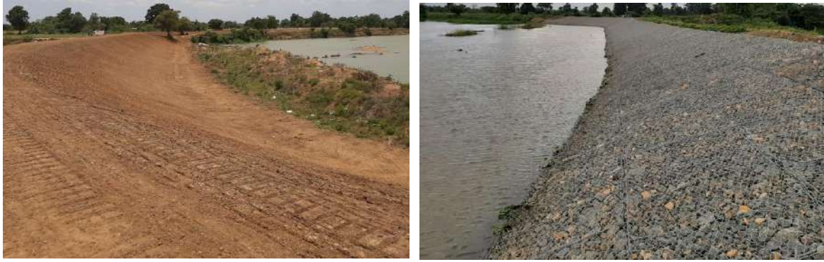
Figure 11-121 Nathanodai Flood Protection Bund
