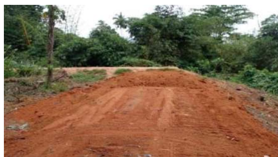
Figure 11-51: Constructed flank bund from 47.2m to 95.3m at Yabalaruwa anicut
