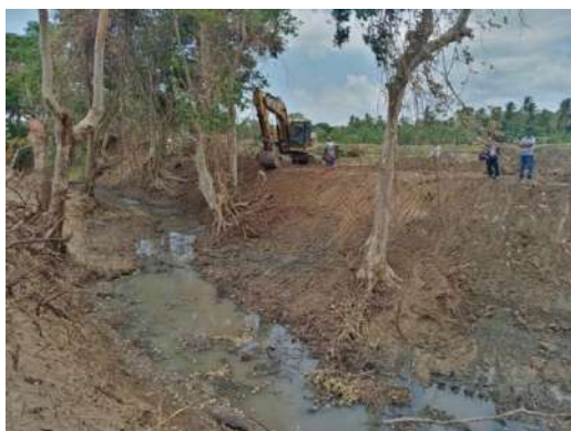
Figure 11-102: Construction of flood bund along Ambagaswewa spill tail canal from 2+790 to 3+900
