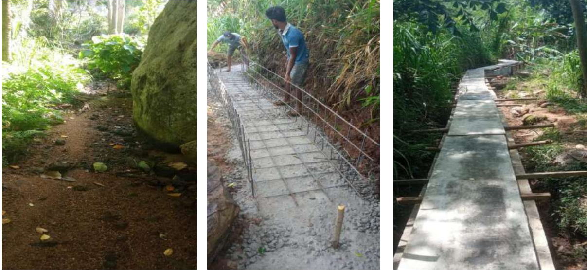
Figure 11-56: Before, during and after construction
