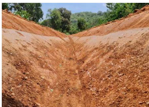
Figure 11-67: Construction of field canals
