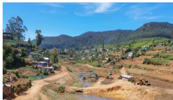
Figure 11-70: Desilting work at Barrack plane tank
