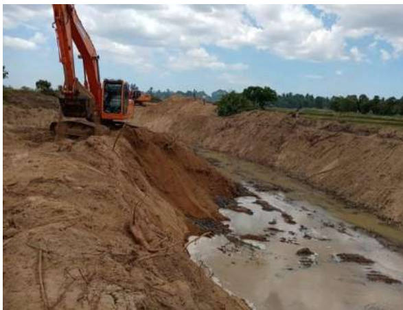
Figure 11-35: Widening and straightening in Mavalai River
