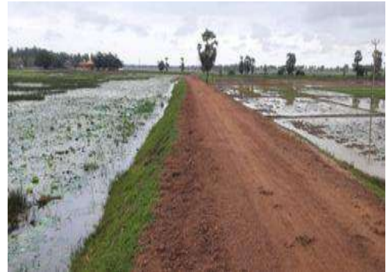
Figure 11-39: Improvements to Vatti Kulam tank bund
