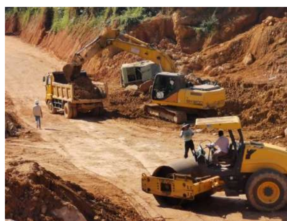
Construction of Roads
