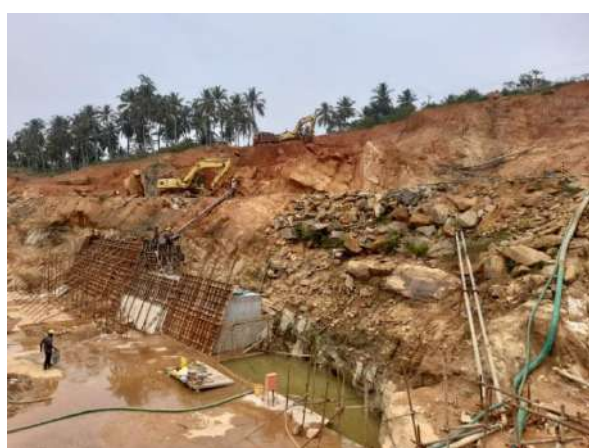
Excavation for core-trench
