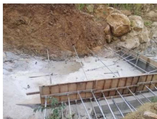
Construction of Saddle Dam
