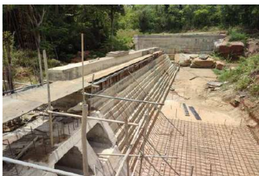
Construction of Anicut
