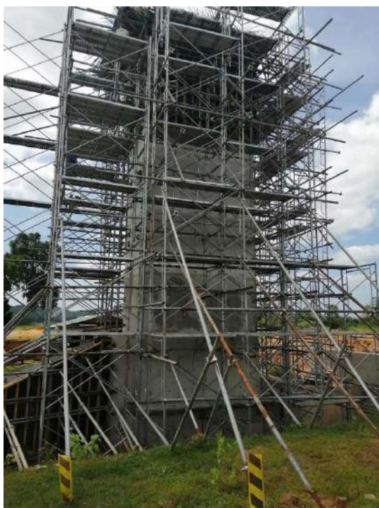
Construction of Sluice Structure
