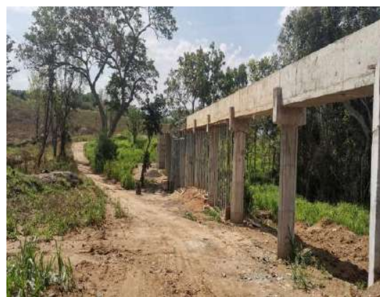
Construction of Structures
