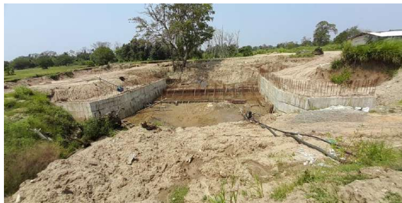
Construction stage of Pan Oya Anicut
