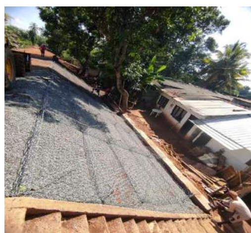
Kelani North Bund Rehabilitation
