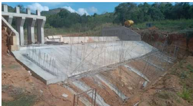
Construction of Spill
