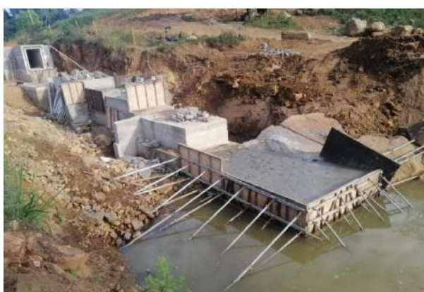
Construction of Sluice Structure
