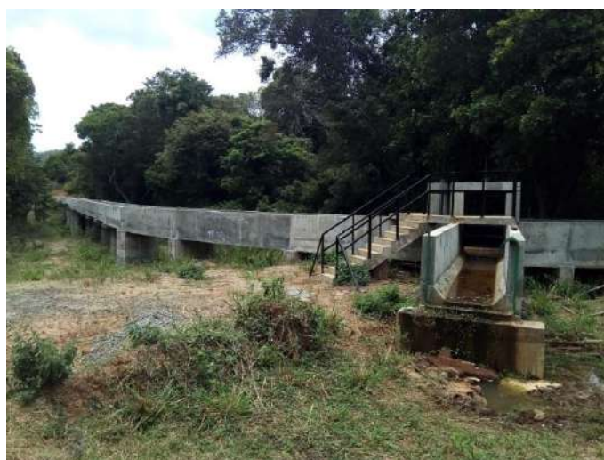
Construction of RB Canal
