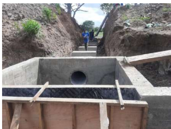
Construction of new sluice
