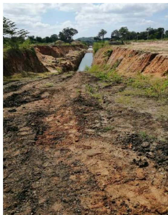
Construction of Dam Axis
