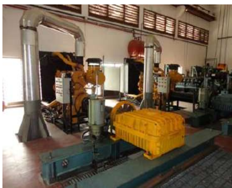
Improvements work - Magallegoda Pump House
