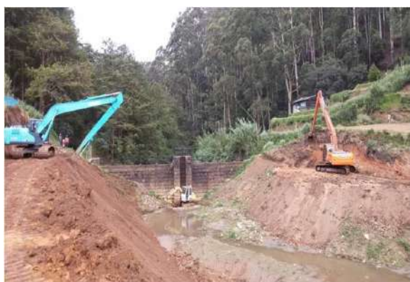
Excavation & Removal of silt in tank
