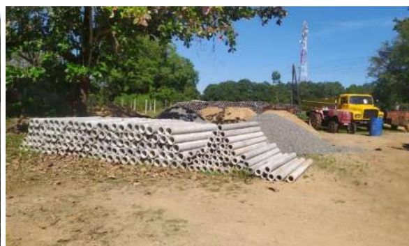
Hume pipes for FTO in Padaviya & Wahalkada Schemes
