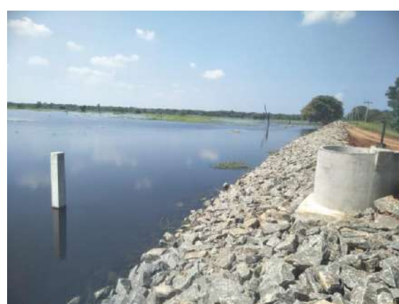
Improvements to tank bund
