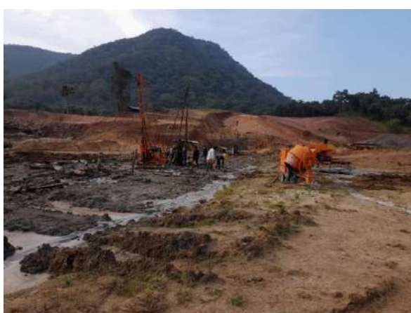
Grouting of Waththedara Tank
