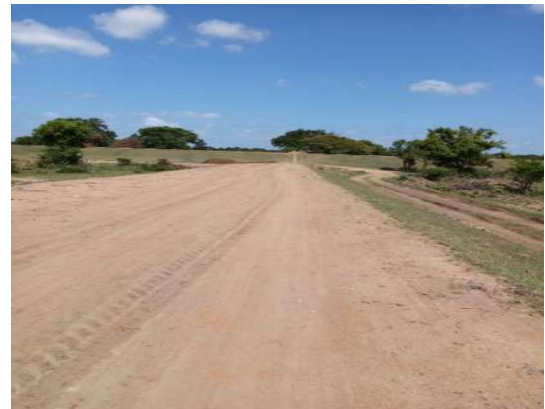
Issanwewa tank bund and MC canal filling
