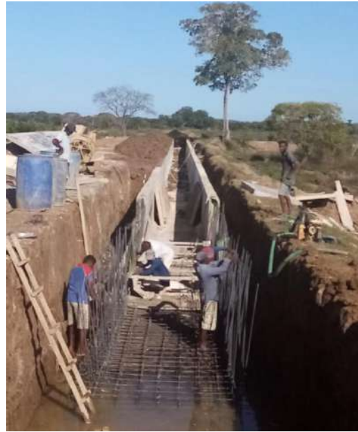
Issanwewa Main Canal
