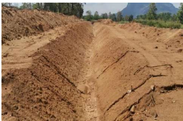
Construction of Main canal
