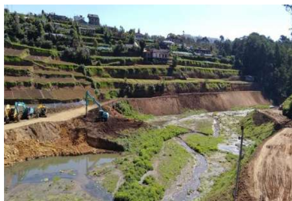
Excavation & Removal of silt in tank
