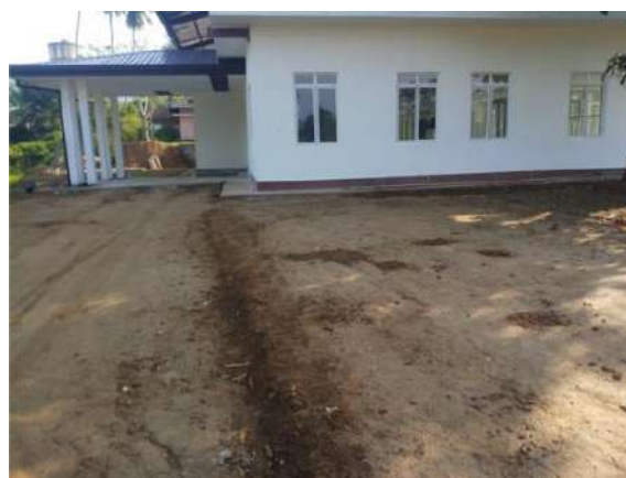
Construction of Project Director's Office
