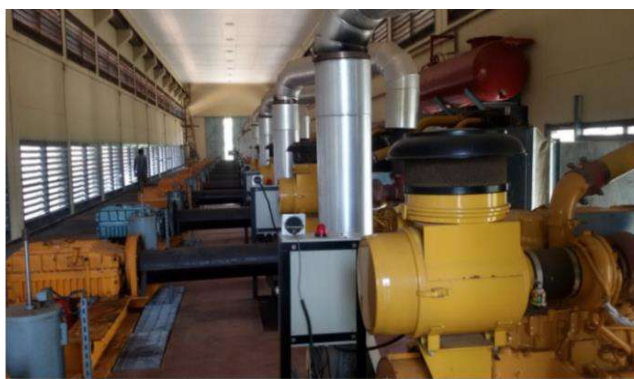
Improvements work - Thalghagoda Pump House
