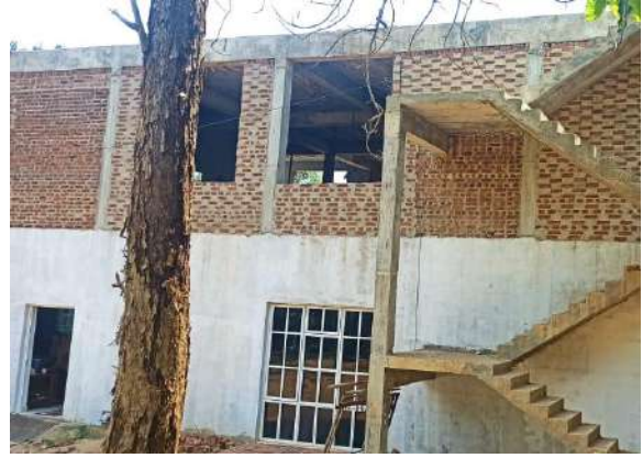
Construction of office building for the PMU and PIU
