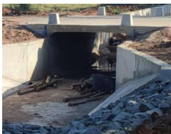
Construction of box culvert
