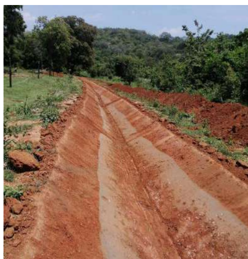
Construction of FC 01
