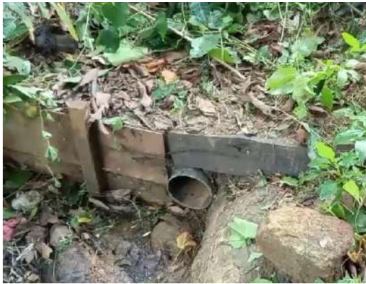
Figure 7: After grouting at section C
