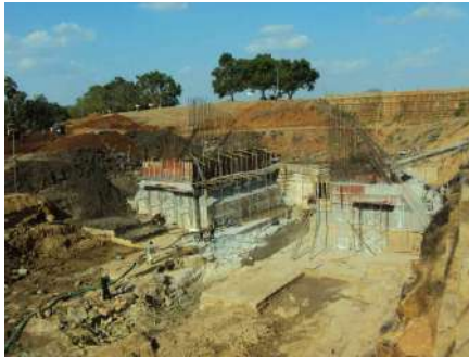
Figure. 12a: A Site View during Construction
