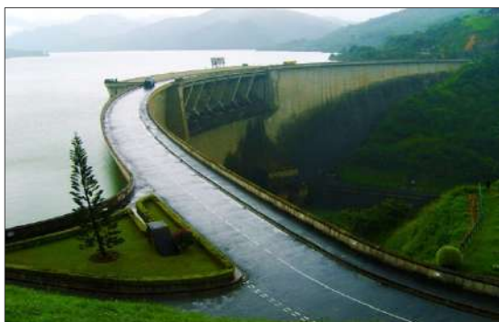
Figure 1: Victoria dam in Sri Lanka.
