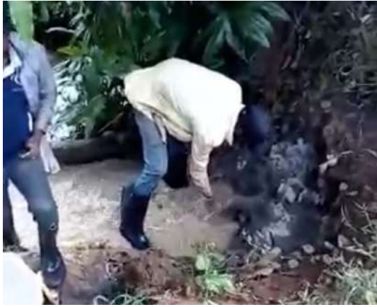
Figure 6: Before grouting at section C
