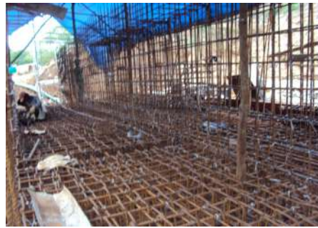
Figure. 12b: Reinforcement Work during Construction
