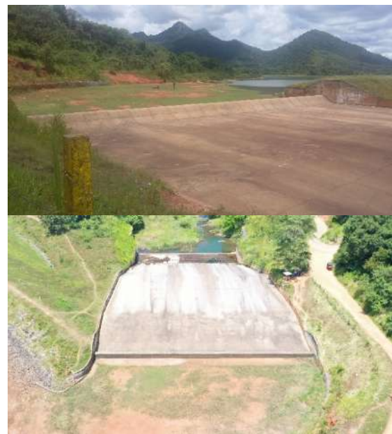
Figure 7: Existing Spillway of Wemedilla Reservoir
