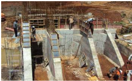
Figure. 12c: Counterforts during Construction
