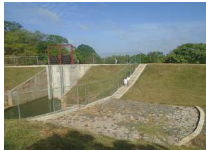
Figure. 12d: A view after the Construction
