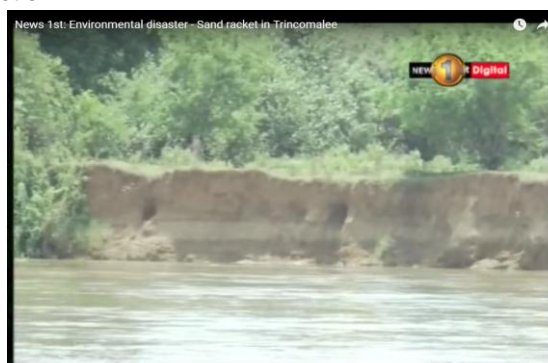
Figure 8 : River Bank erosion due to mining in the Mahaweli at Trincomalee
